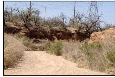
Deep headcutting causing loss of native vegetation along the river corridor
