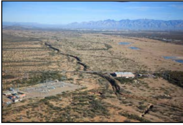
Head-cut Santa Cruz River channel extending south past Pima Mine Rd.
