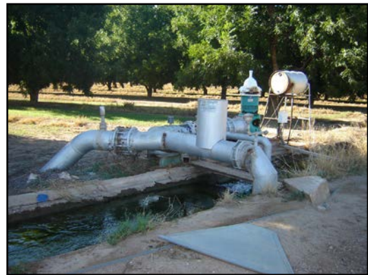
Existing groundwater well
