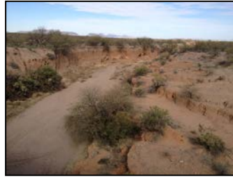
Deep, narrow, unstable channel at Pima Mine Rd. due to headcutting.
