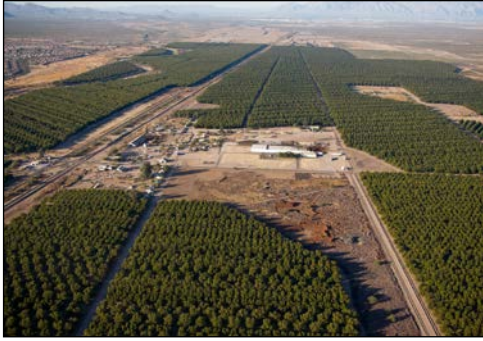
Existing Site Conditions
